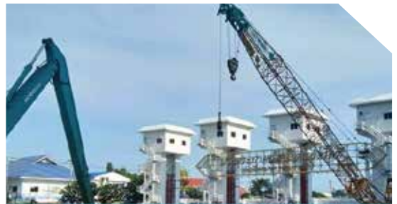
Bank protection wall at Klong Lat Pho Floodgate project, Samuthprakarn
