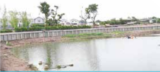
Bank protection wall project, Property Perfect PLC, Pathumthani.
