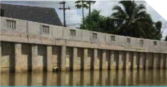
Flood protection wall project, Kraburi, Ranong.
